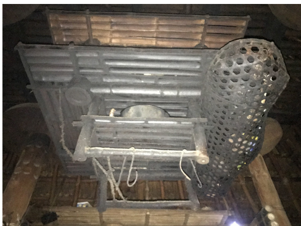
Figure 6. The material regeneration process through weathering of the bamboo surfaces (left) and the blackening of the material above the hearth (right) (Photographs by authors)
