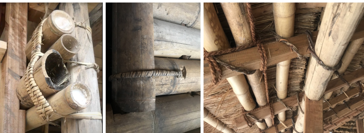
Figure 5. Types of Sumbanese traditional joinery: rattan joinery (left), combination of rattan and pegs joinery (middle), and the combination of coconut fibre and roots joinery (right) (Photographs by authors)
