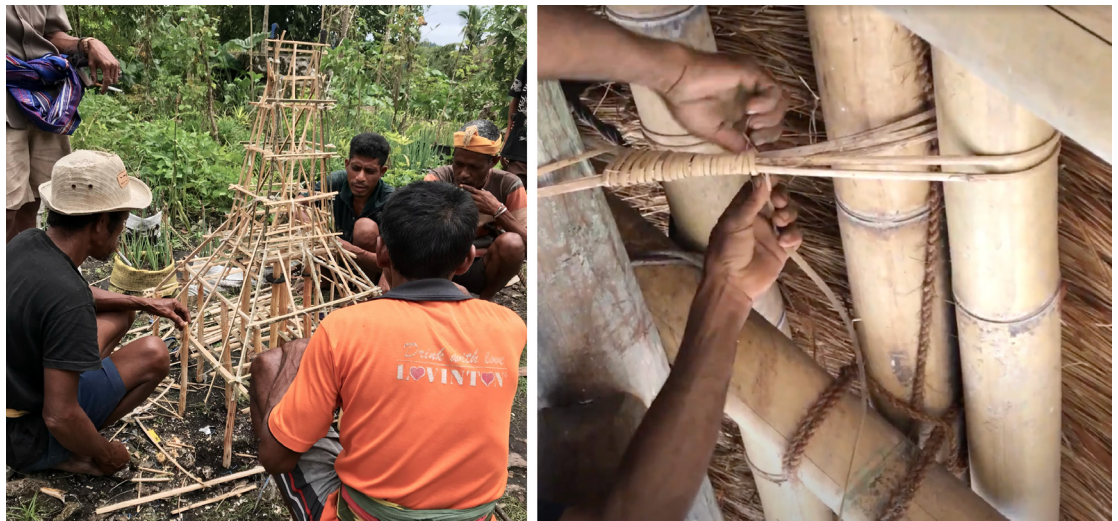
Figure 3. Demonstrations of the construction process by the community during the field study, including building a maquette (left) and the rattan tying technique (right) (Photographs by authors)
