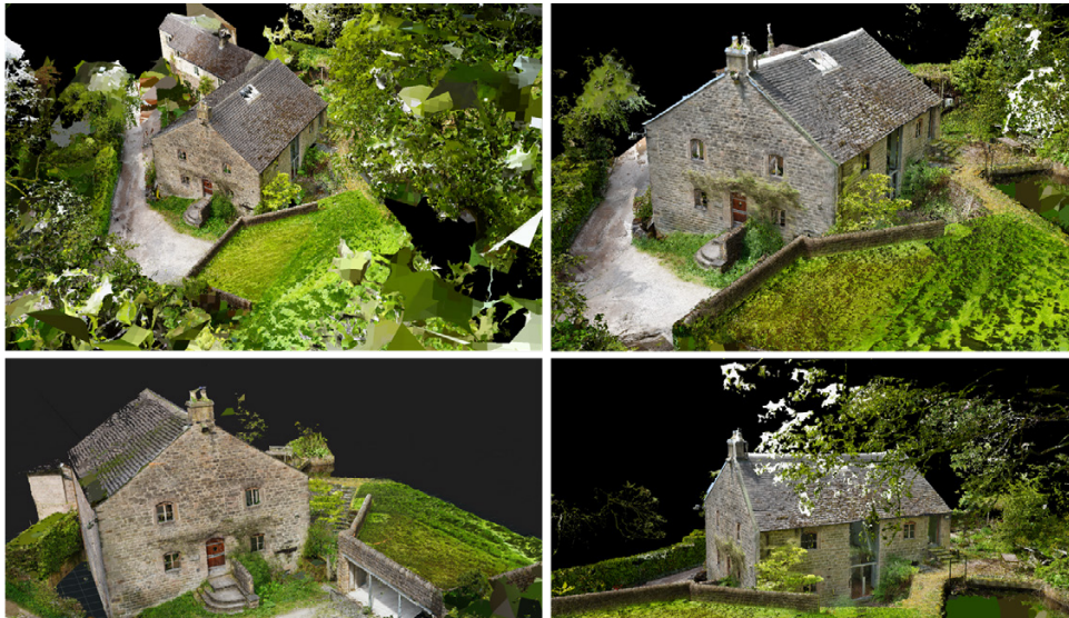
Figure 16. Aerial perspectives on the relationship between the building and landscape generated from the 3D scanning model (Images by authors)
